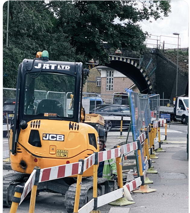
Less excavation means less inconvenience for the general public.
