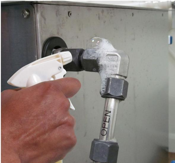
An easily identifiable bubble at a leaky connection
