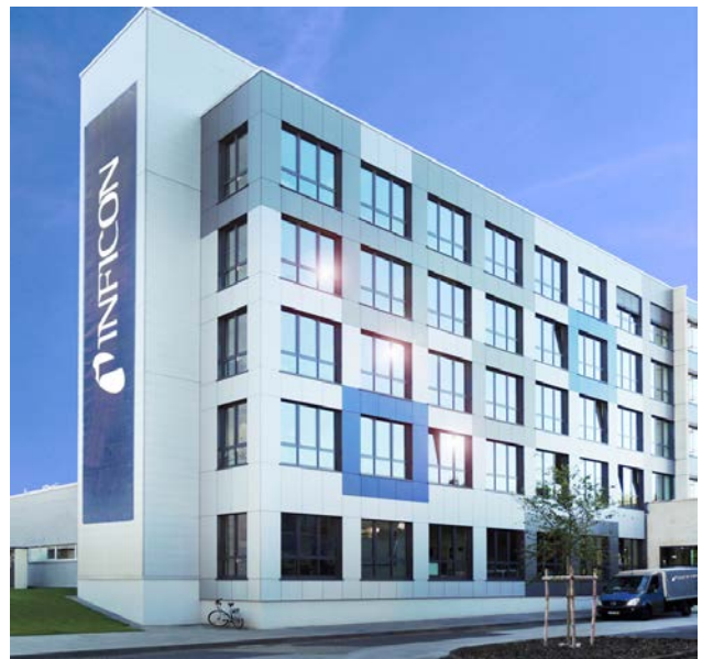
INFICON production facility in Köln, Germany – development, design and manufacturing of leak testing production tools
