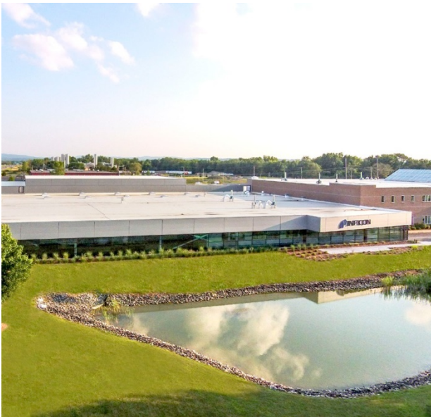
INFICON production facility in Syracuse, NY – development, design and manufacturing of leak detection service tools
