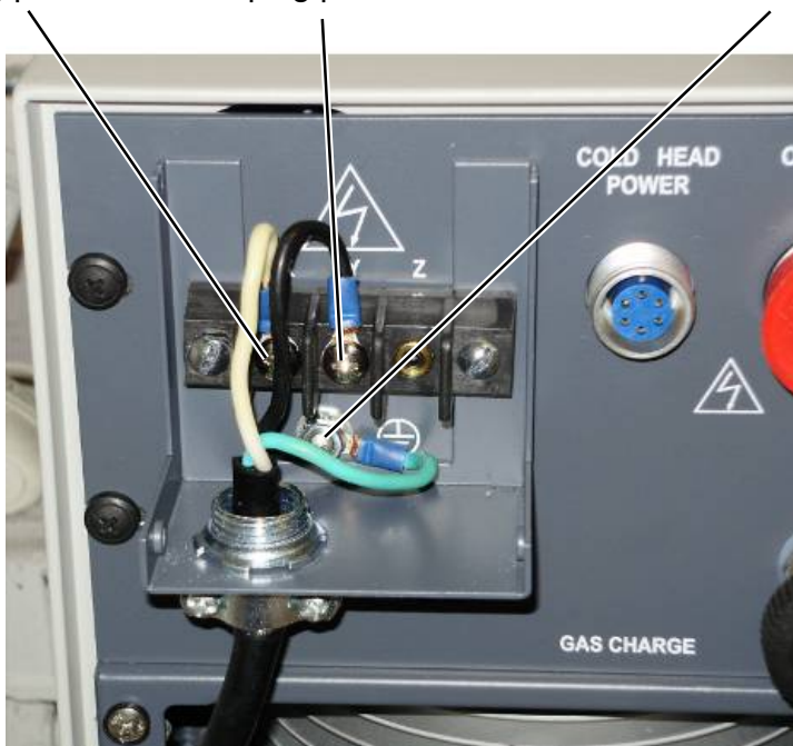
Fig. 10: Compressor: Terminal points for the connection of the power cord
