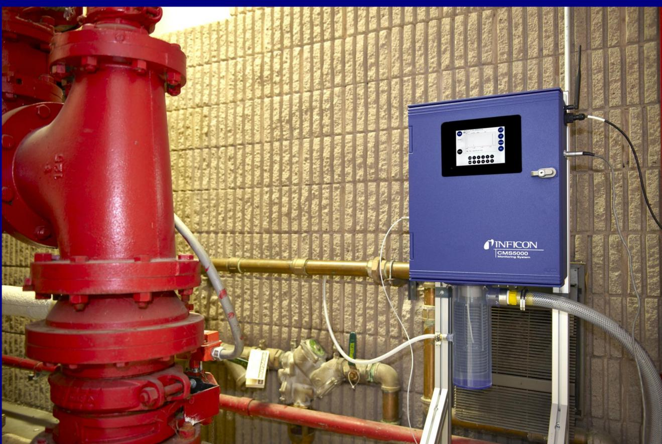
Figure 1: CMS5000 configured for continuous water monitoring
